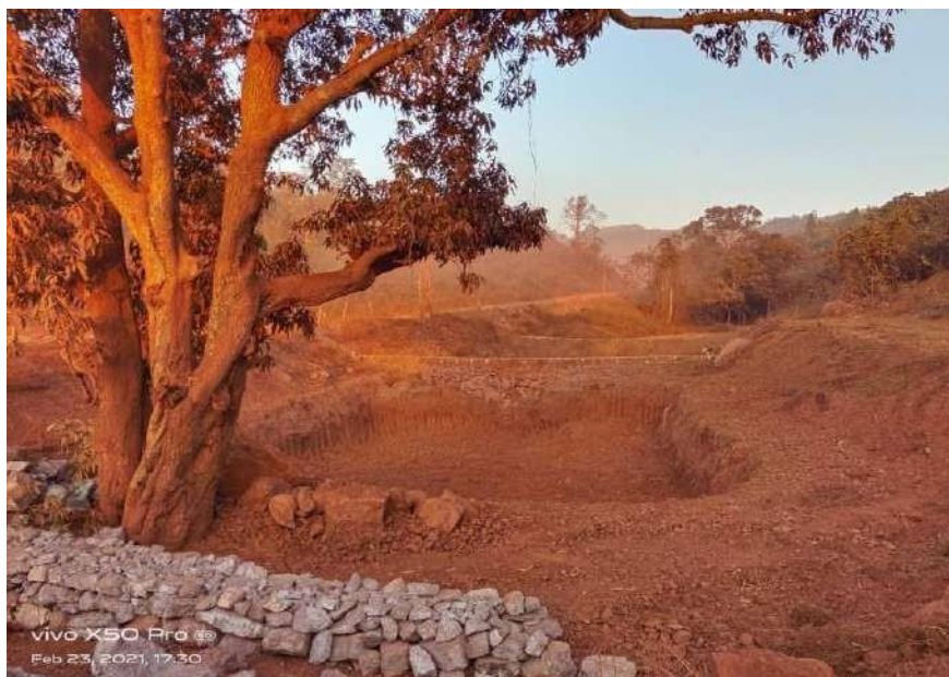
Series of Settling Ponds
